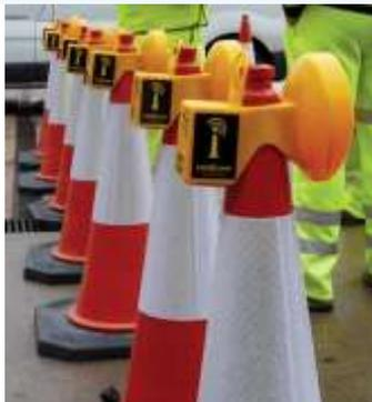
Creating safer workzone environments is "intellicone" from the UK; if one cone is displaced a signal is sent to all other "intellicones" around the zone, with alert siren and flashing beacons.
