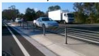
Four strand, steel rope barriers have proved very effective (although our Motorcycle Council of NSW have voiced their concerns) when deployed with sufficient run-off, due to the deflection properties of the barrier.
