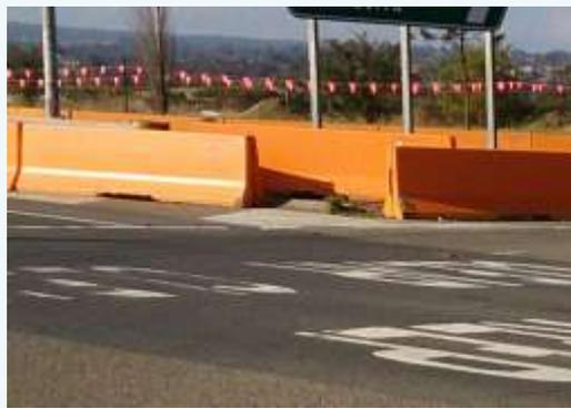
Disregarding my personal views towards temporary concrete barriers, the following slide displays a concrete barrier with signs of surface spalling and the other, painted concrete barriers. I may have been misinformed but I understood that painting was not permitted so that issues such as spalling or patching could be clearly identified?
