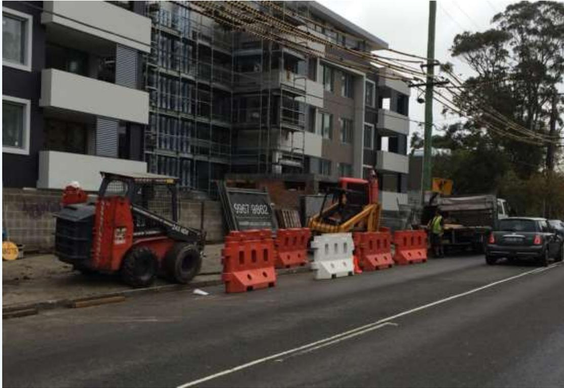
Obviously it is imperative that safety technologies are deployed corresponding to the manufacturers' specifications. As you can see from this particular instance, that is not always the case. You may judge for yourself as to whether these barriers were even filled with water.
