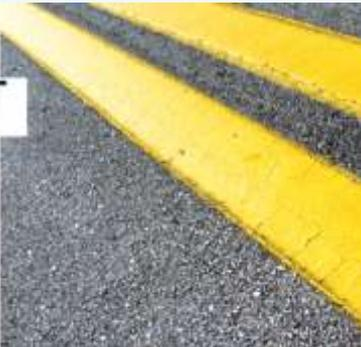
A directional line marking trial has recently been undertaken in Victoria for workzones where existing markings have been left in-situ but additional double yellow lines have been applied to give direction. A simple but interesting concept designed to avoid ghost marking through sun glare and presumably the cost of white-line removal and replacement as the yellow lines are degradable.
