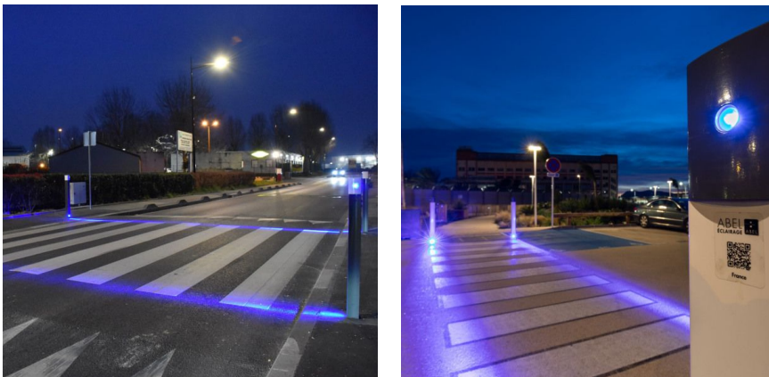
Figure 2 – Examples of Wattway installations
