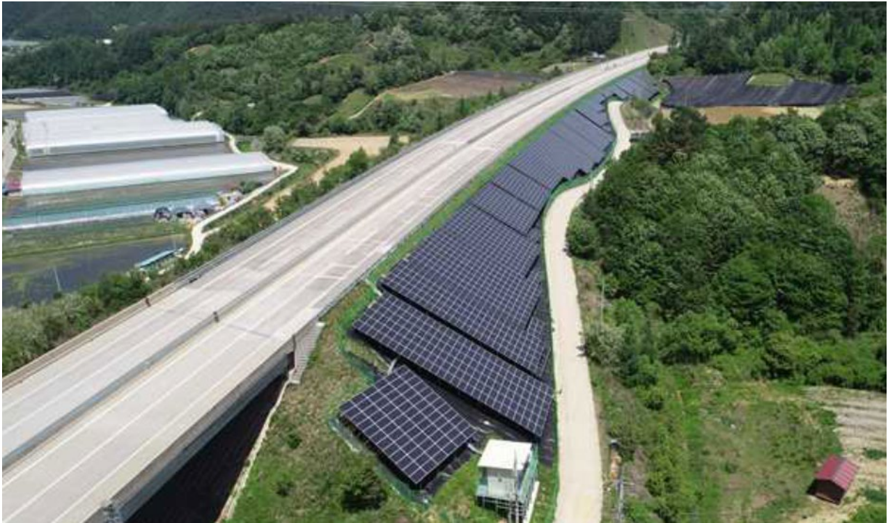
Figure 8 - An example of a solar microgrid adjacent to freeway in South Korea (Bellini, 2021).
