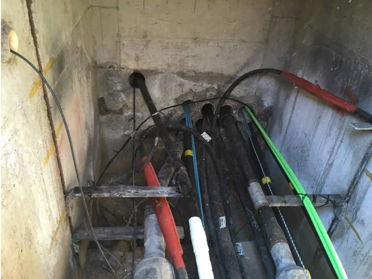
Figure 11 Construction Example of Major Telecommunications Pit
